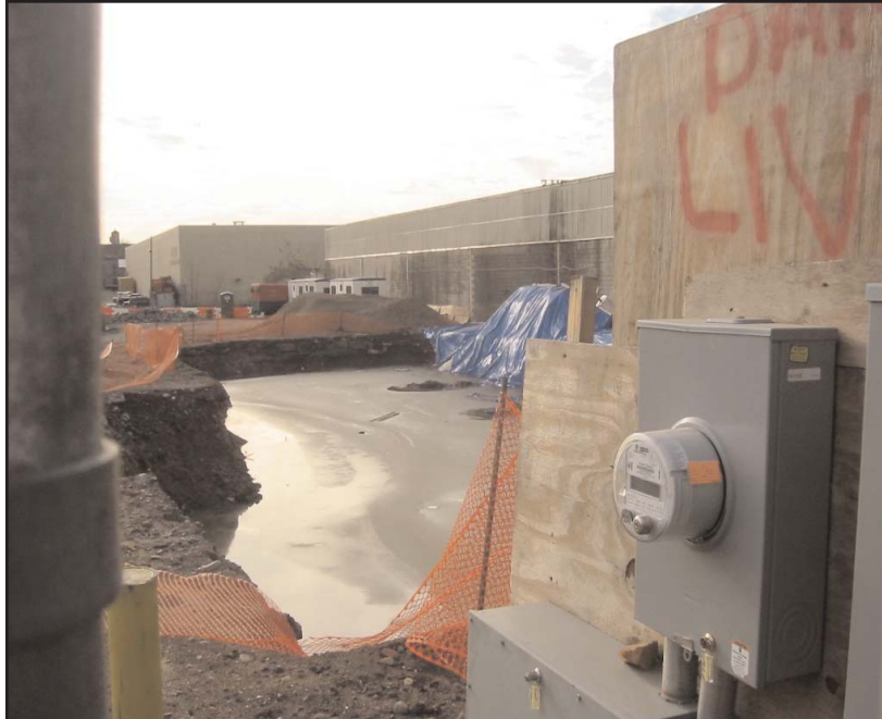
Brownfield remediation is currently underway along the canal near Third Street on the property that the proposed Whole Foods will occupy.
